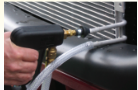
The convenient return hose allows easy management of used flush.
